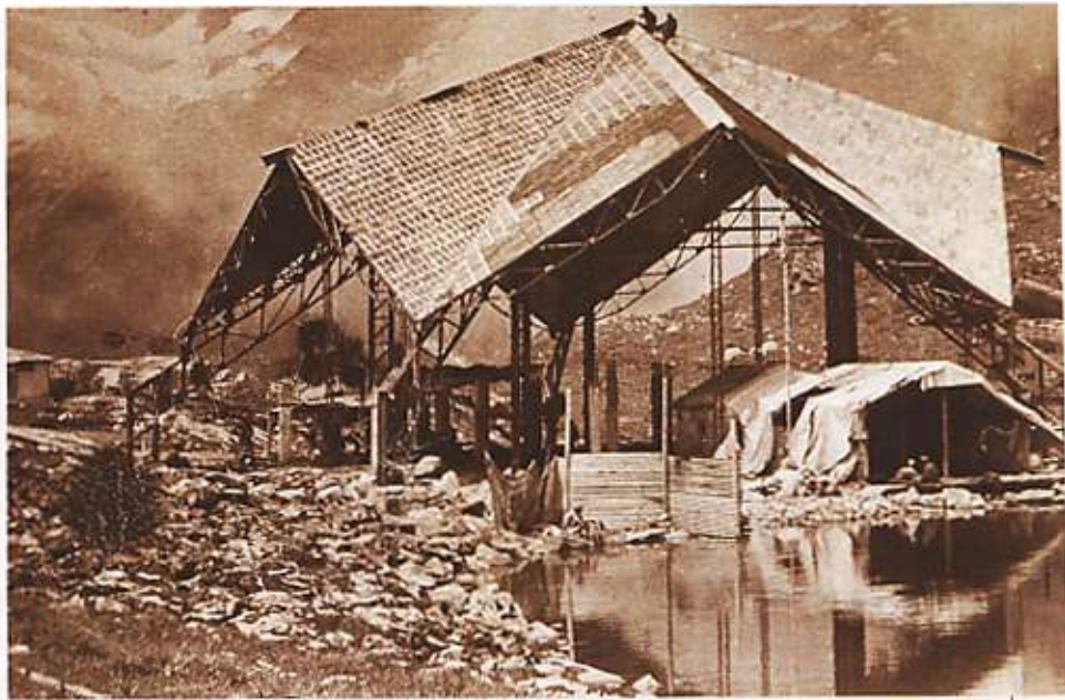
Boarding of astrolite, being laid over steel trusses in 1974.
