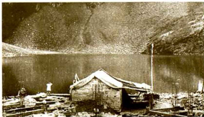
To conserve the old Gurdwara which was constructed in November 1935 with local materials, structure of the new Gurdwara was so placed that the old became part and parcel of the new, falling under the valley truss, towards the lake side.
