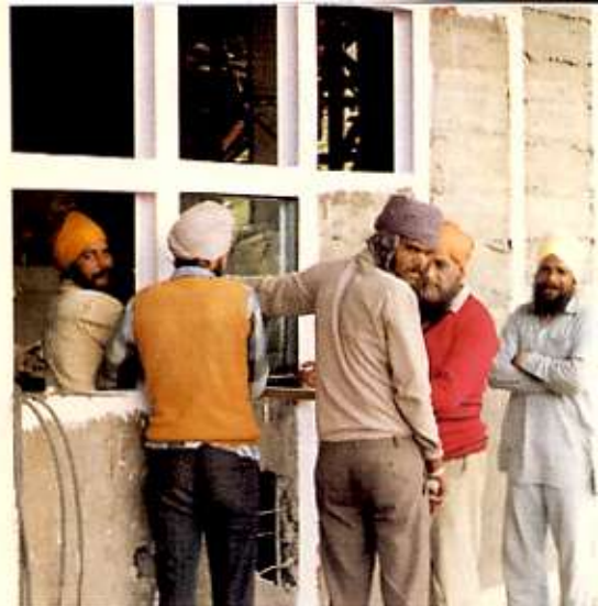
Glazing being done along the corridor.
