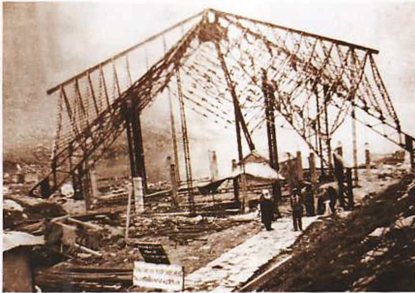
Erection of the steel structure over the old Gurdwara building.
