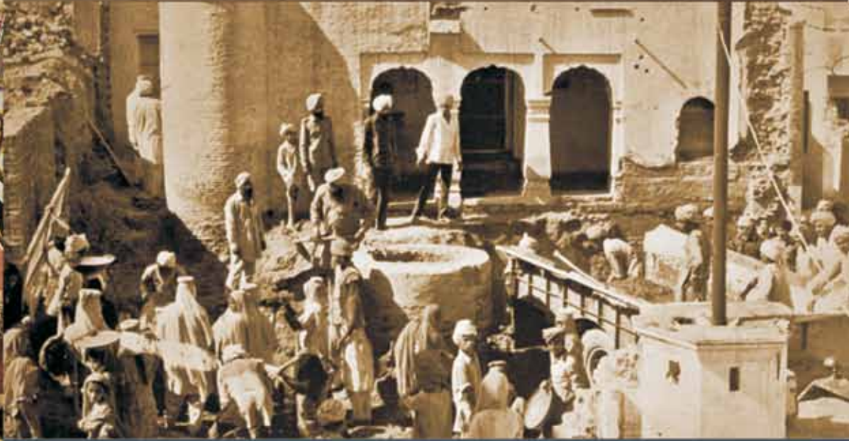
A VIEW OF THE DEMOLITION WORK BEING CARRIED OUT BY KAR SEVAKS AT THE OLD GARHI SAHIB GURDWARA.
