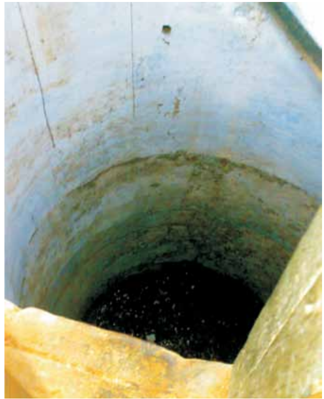
The well in the bagh.
