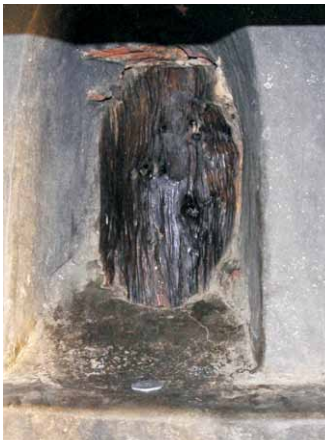
Wooden pillar, piled into the ground as foundation of the village.
