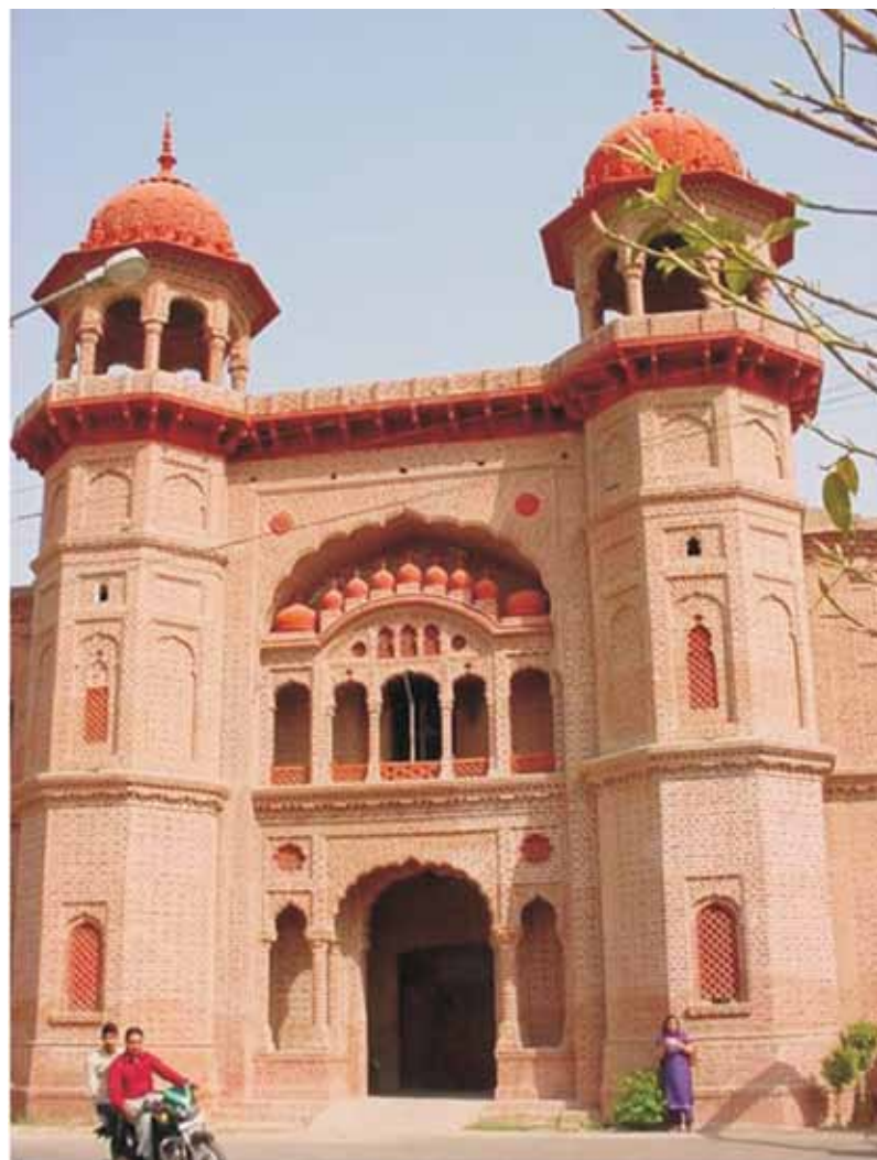
Khalsa College Amritsar; entrance to the Boarding House.
