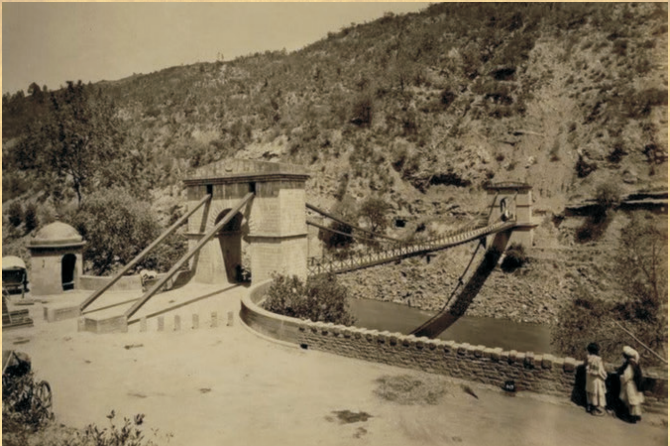
Kohala Bridge over the River Jhelum, connecting the north west frontier and Kashmir
