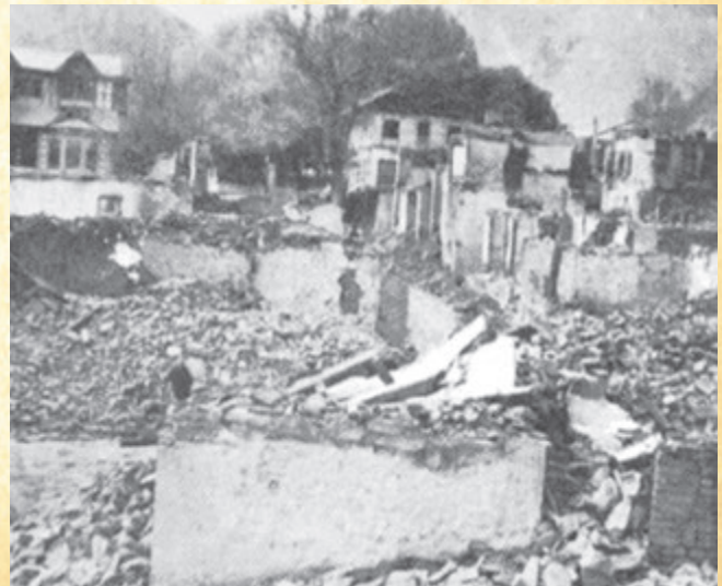
Destruction of Baramula after pillaging and arson by the Kabalees
