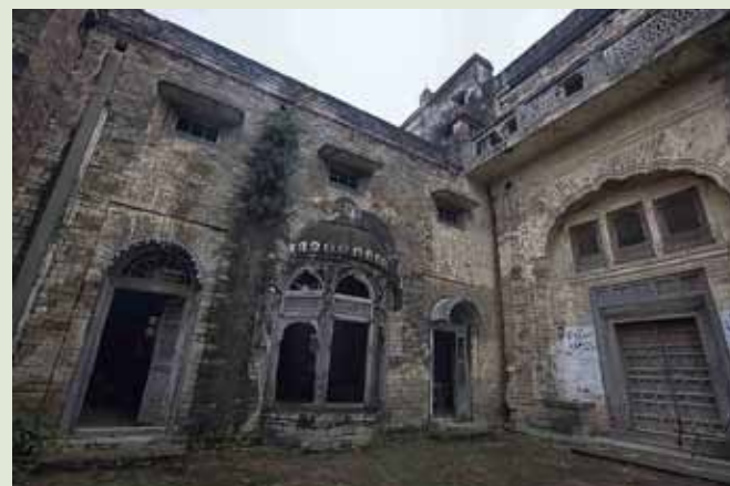
Finely crafted doors and windows of the Bedi haveli
