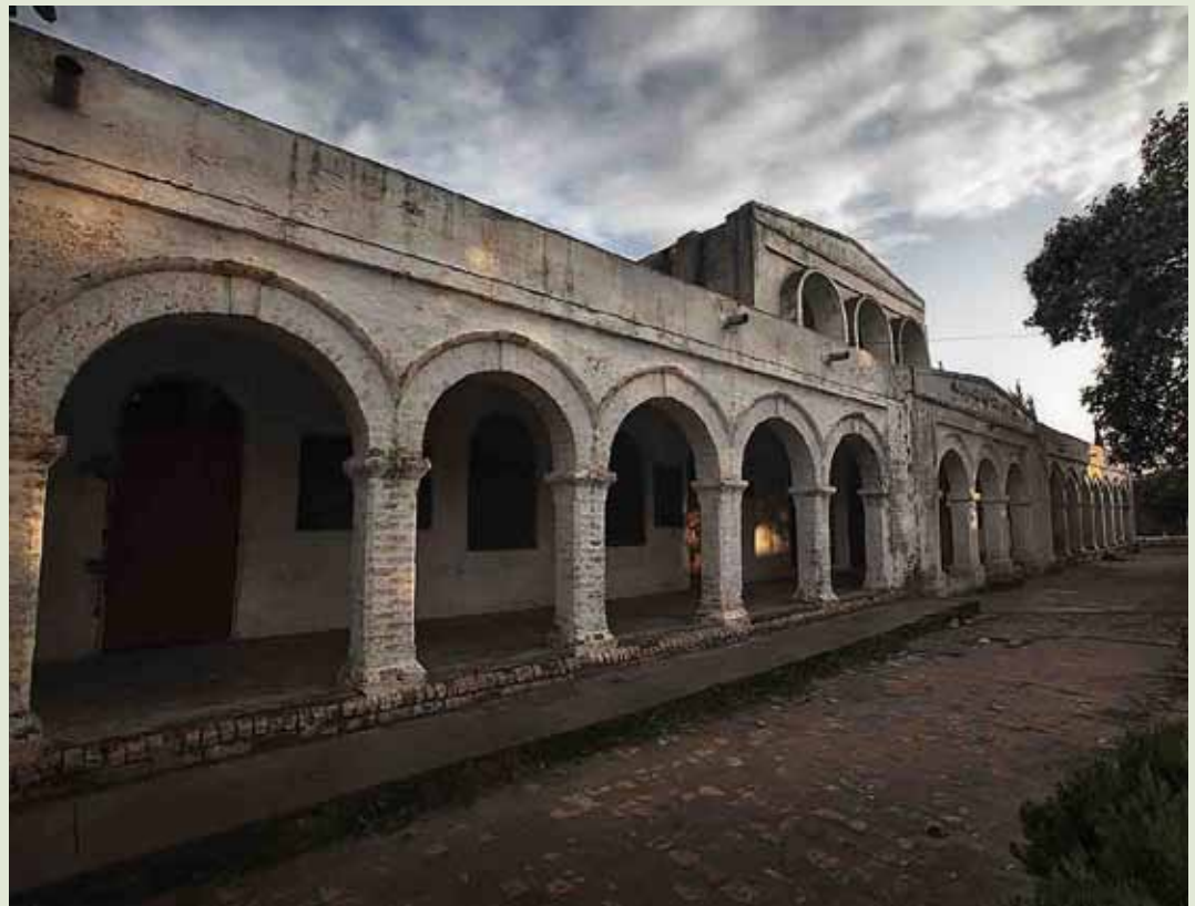
Classroom wing of the Khalsa School at Saagri village
