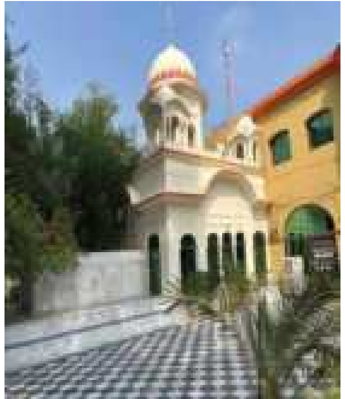
Gurdwara Beri Sahib, Sialkot after Restoration
