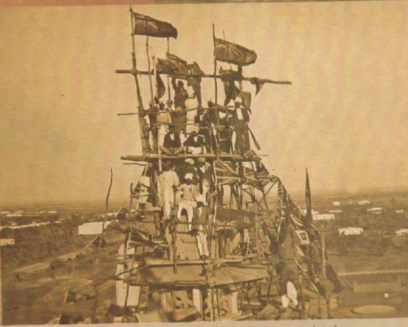
Atop the South Block, which was completed on 30 September 1927, are the engineers and workers who 'won' the race against the North Block !
