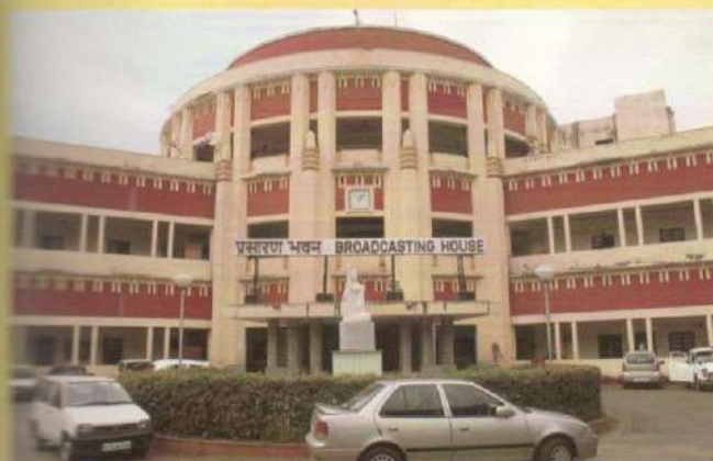
All India Radio Building
